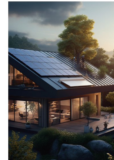
Residential Photovoltaic Energy Storage
