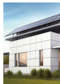
Residential Photovoltaic Energy Savings
